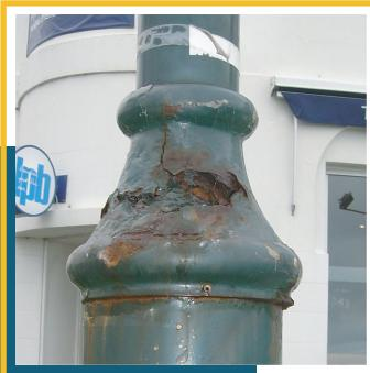
The joints are not sealed from the weather, so water running down the pole gets trapped behind the decorative spinning, causing premature corrosion.
